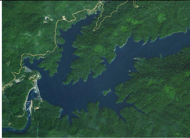
Figure 8.16(a, b): Gerusoppa dam Project area
