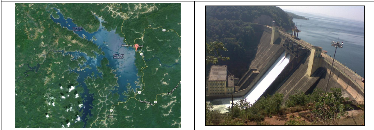
Figure 8.4 (a, b): Supa dam Project area
