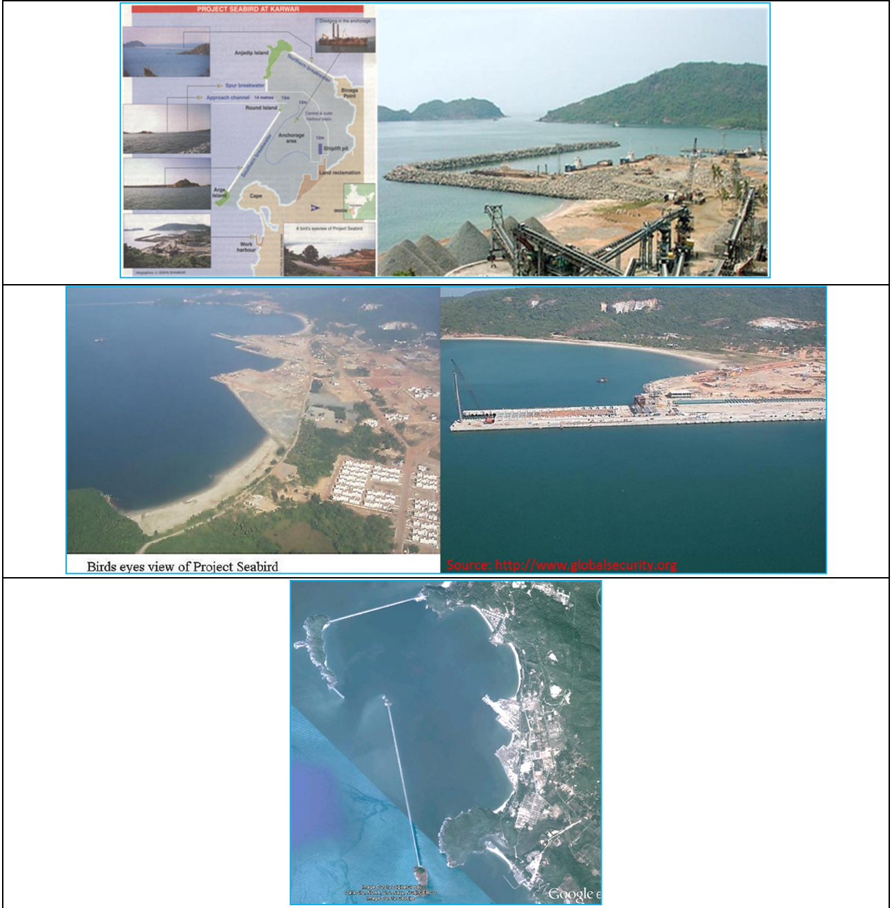
Figure 8.19: the location of Project seabird as shown in Google Earth and other
